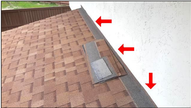
Item 1 - Item- (Picture 1) No evidence of proper flashing
