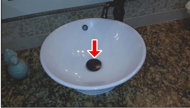
Item 36 - Item- (Picture 1) Drain stop is stuck
