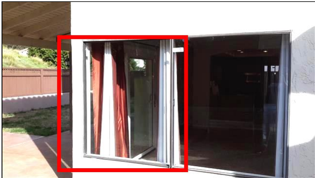
Item 7 - Item- (Picture 1) No window screens installed
