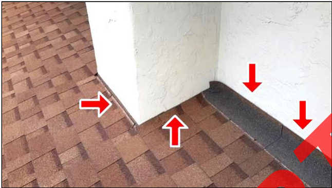
Item 1 - Item- (Picture 2) No evidence of proper flashing
