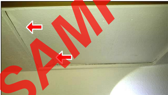
Item 4 - Item- (Picture 1) Attic access panel is cracked/damaged
