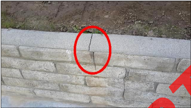
Item 9 - Item- (Picture 7) Small crack
