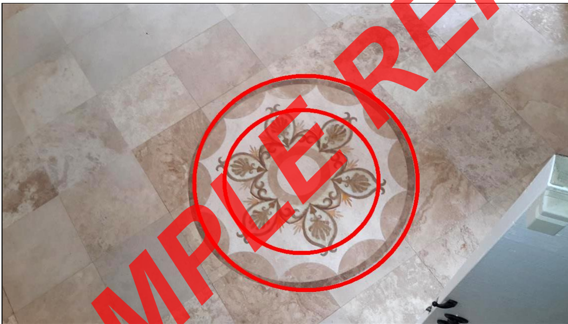
Item 38 - Item- (Picture 2) Center circular tile is hollow
