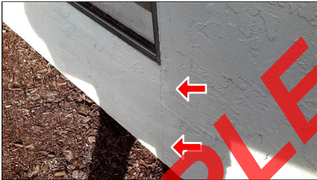
Item 5 - Item- (Picture 6) Small exterior crack
