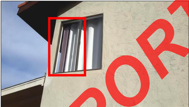
Item 7 - Item- (Picture 2) No window screens installed
