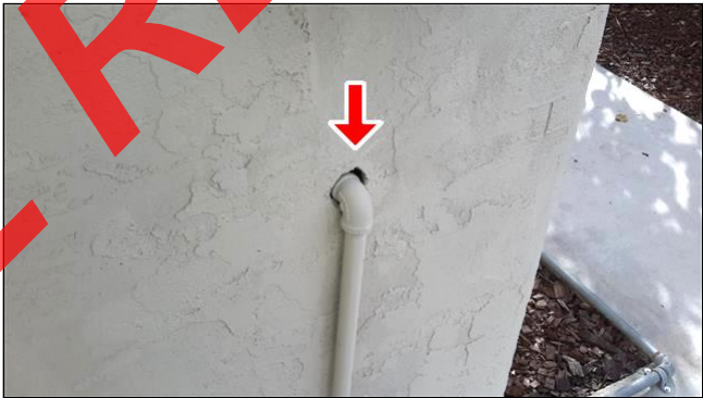
Item 5 - Item- (Picture 7) Pipe and stucco not sealed
