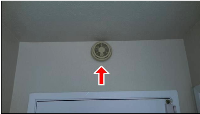
Item 43 - Item- (Picture 1) Does not operate when tested
