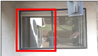
Item 7 - Item- (Picture 3) No window screens installed
