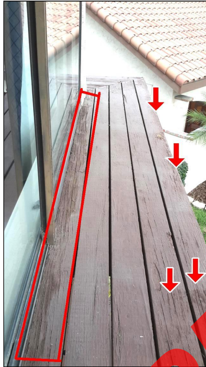
Item 8 - Item- (Picture 2) Wood Rot Damage
