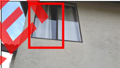
Item 7 - Item- (Picture 5) No window screens installed
