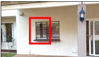
Item 7 - Item- (Picture 8) No window screens installed
