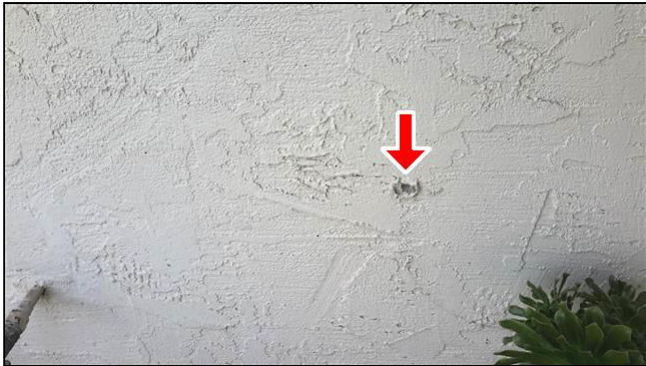
Item 5 - Item- (Picture 5) Small hole in the stucco
