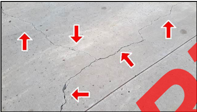
Item 9 - Item- (Picture 3) Small cracks
