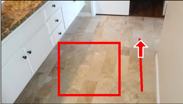
Item 38 - Item- (Picture 1) Loose tile and floor slats slightly
