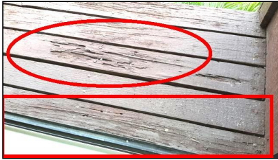
Item 8 - Item- (Picture 1) Wood Rot Damage
