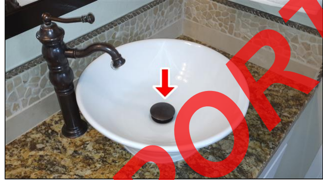
Item 36 - Item- (Picture 2) Drain stop is stuck
