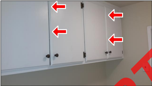
Item 17 - Item- (Picture 2) Doors bind when closing
