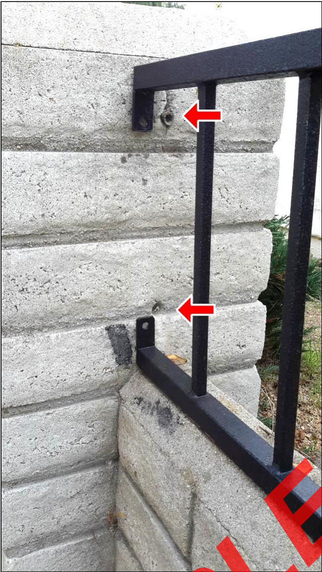
Item 9 - Item- (Picture 6) Missing bolts to railing
