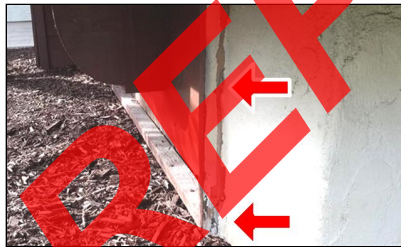
Item 5 - Item- (Picture 2) Wood rot & wood exposed
