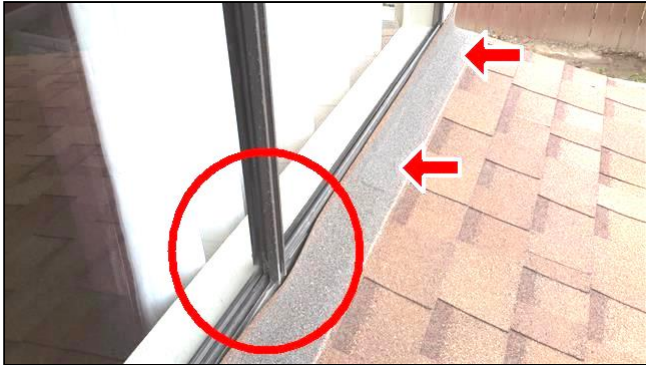
Item 1 - Item- (Picture 3) No evidence of proper flashing
