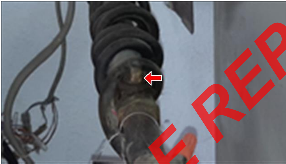
Item 41 - Item- (Picture 1) Furnace Gas Shut-Off Valve is not a manual turn
