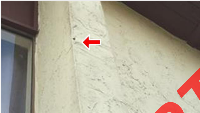
Item 5 - Item- (Picture 4) Small hole in the stucco
