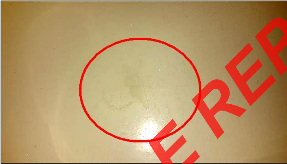
Item 33 - Item- (Picture 3) Small cracks in the tub finish
