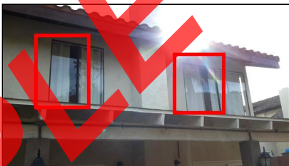
Item 7 - Item- (Picture 7) No window screens installed
