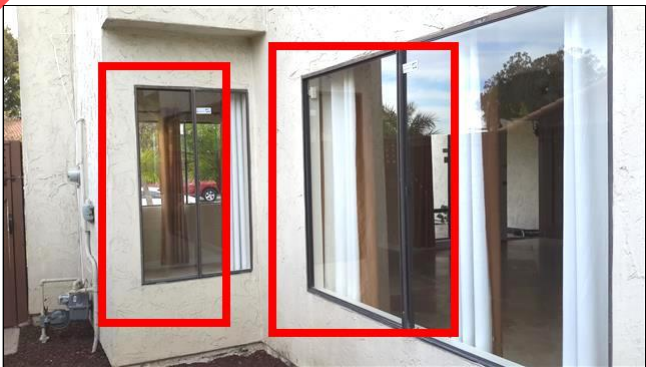
Item 7 - Item- (Picture 10) No window screens installed
