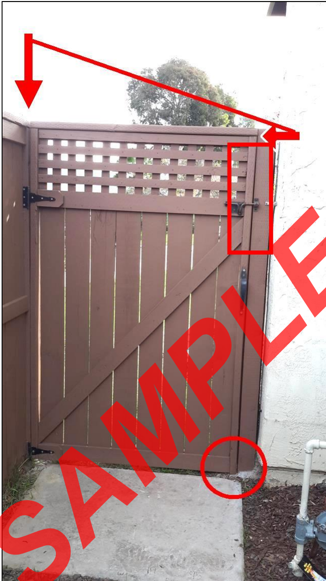
Item 9 - Item- (Picture 10) Gate heavy causing gate to rub
