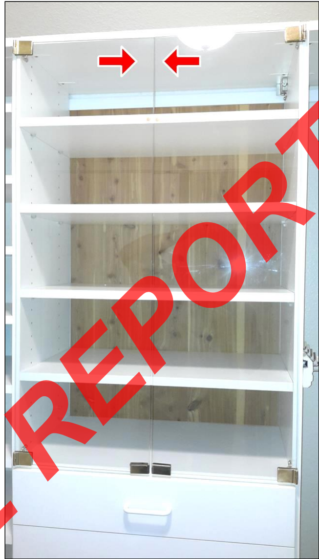
Item 34 - Item- (Picture 2) Glass doors bind when closing
