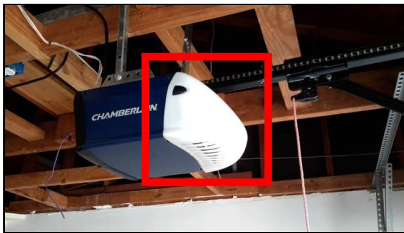
Item 12 - Item- (Picture 1) Light to single door does not work
