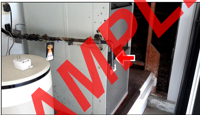
Item 41 - Item- (Picture 2) Sediment trap not installed properly
