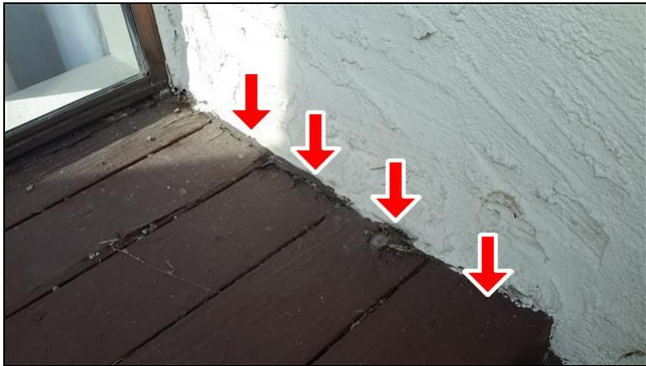
Item 5 - Item- (Picture 3) Wood ledge dry rotting
