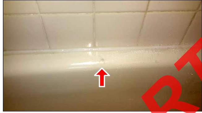
Item 33 - Item- (Picture 2) Small chip in the tub
