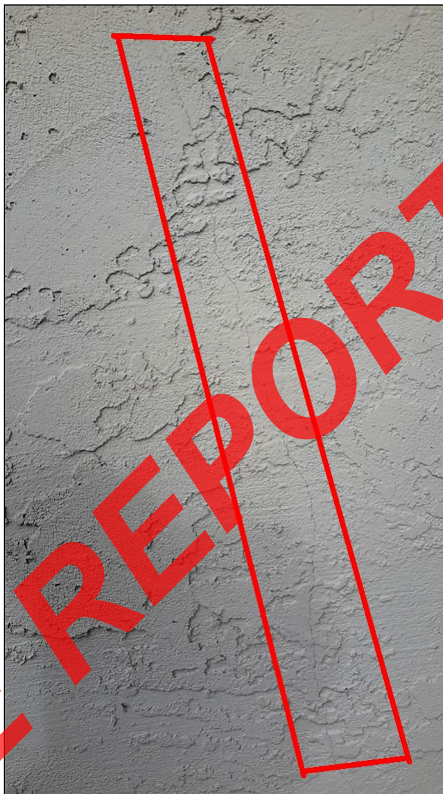
Item 5 - Item- (Picture 9) Small crack in stucco wall
