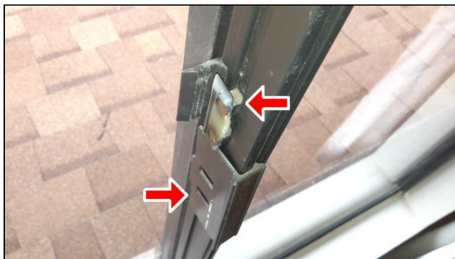
Item 25 - Item- (Picture 1) Window lock broken
