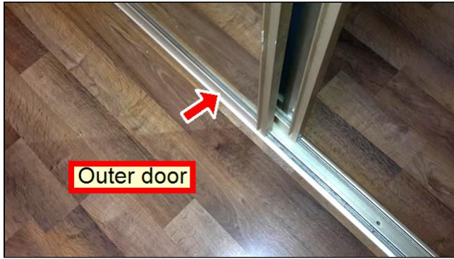
Item 23 - Item- (Picture 1) Door caster wheels worn/ broken
