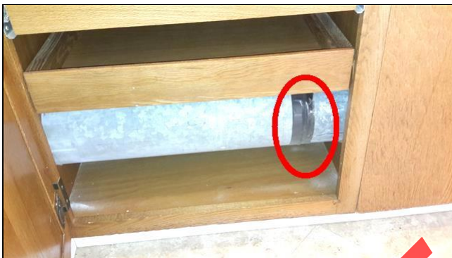
Item 15 - Item- (Picture 1) Incorrect ducting tape
