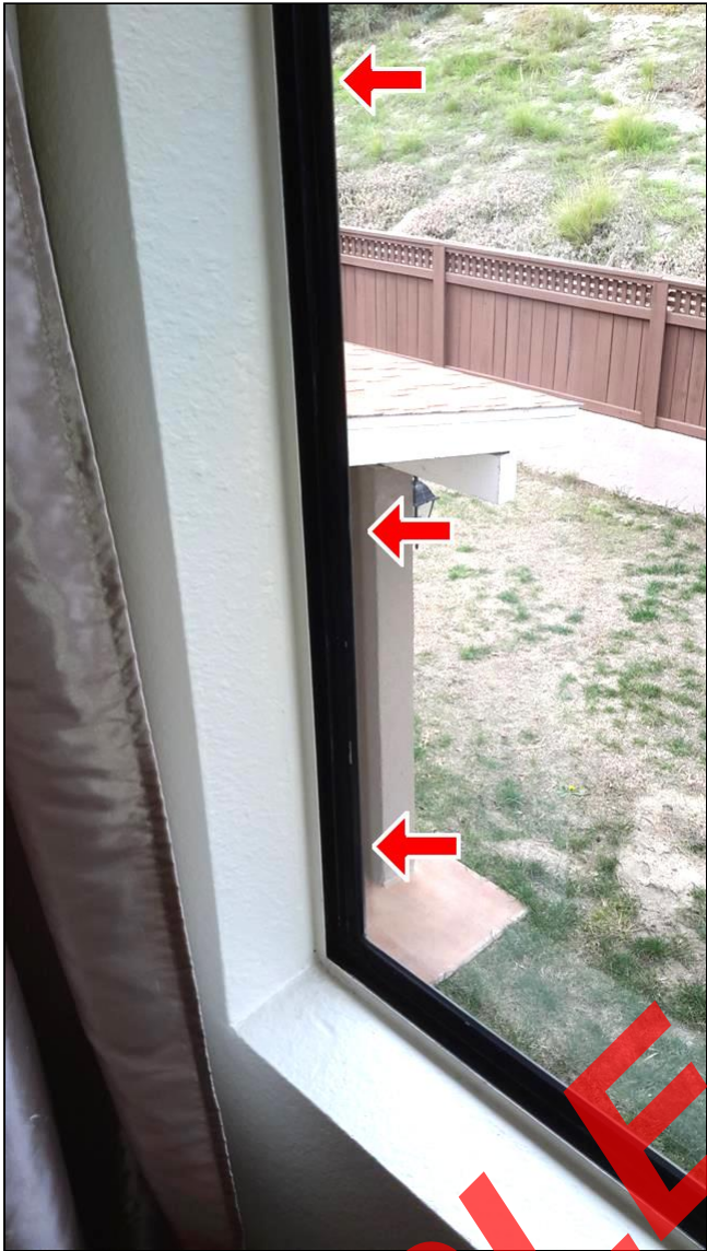
Item 27 - Item- (Picture 1) Window shakes within the frame (Loose)
