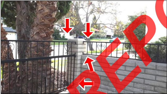
Item 9 - Item- (Picture 5) Loose metal fencing
