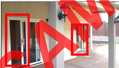
Item 7 - Item- (Picture 9) No window screens installed
