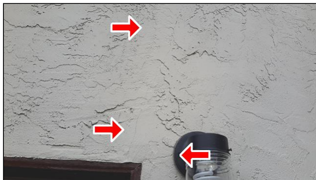
Item 5 - Item- (Picture 8) Small crack in the stucco
